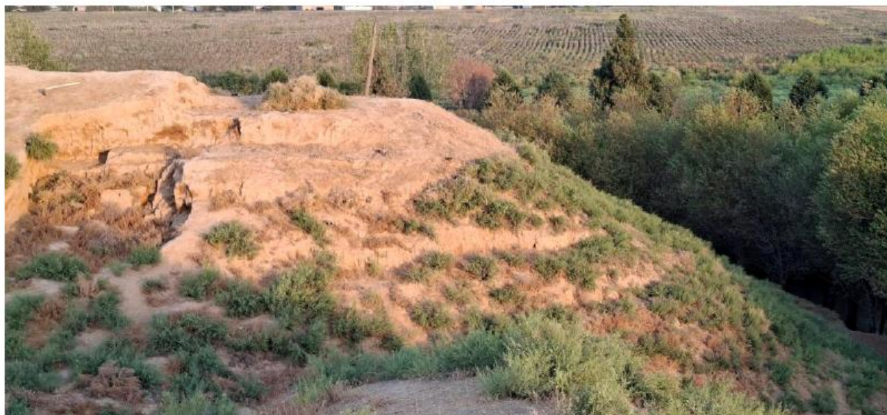
Figure 7. Condition of the northern tower prior to excavation
