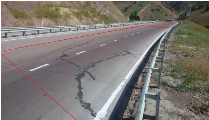
Rice. 1. The results of the negative impact of the movement of trucks with overload on the roads of the Republic of Uzbekistan
