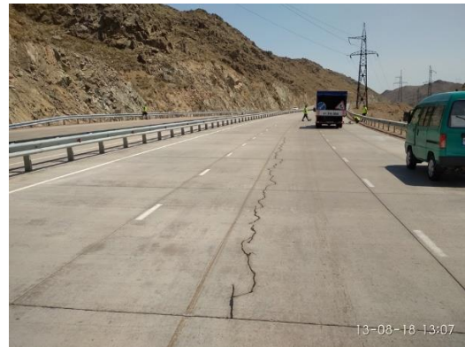
Rice. 1. The results of the negative impact of the movement of trucks with overload on the roads of the Republic of Uzbekistan
