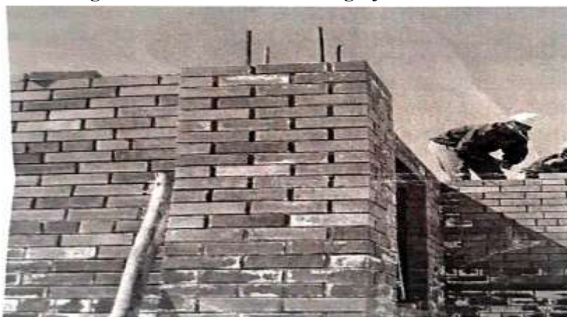
Figure 2. Exterior wall corner with monolithic reinforced concrete columns made of brick in a residential building (Navoi city).
