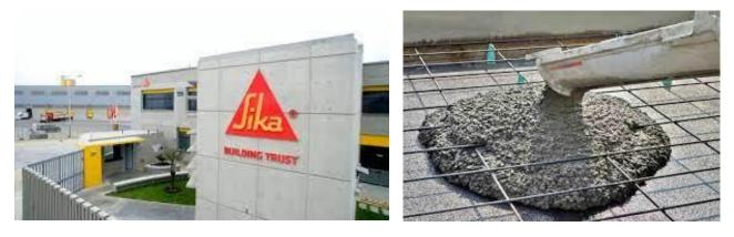
Reducing the water-cement ratio in concrete mixtures is relevant, because if more water is added to the concrete mixture than the norm, the more pores there will be in the hardened concrete structure. These pores reduce the strength and frost resistance of concrete. This is due to the fact that in winter, if water enters the pores and freezes (water expands by about 9%), the overall structure will be damaged.
